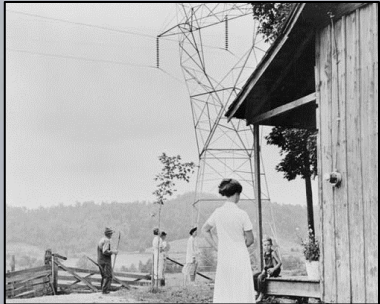
The meter on the wall of the rural shack shows that it now receives electricity.
