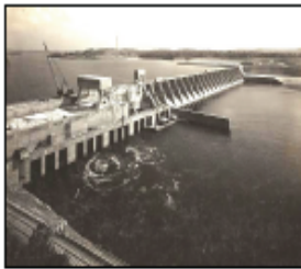
Watts Bar dam on the Tennessee River
