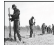
CCC workers putting up a fence in Greene County, Georgia (1941)
