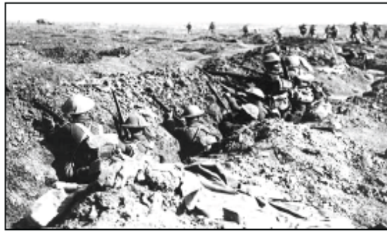
Soldiers used trenches for protection.
